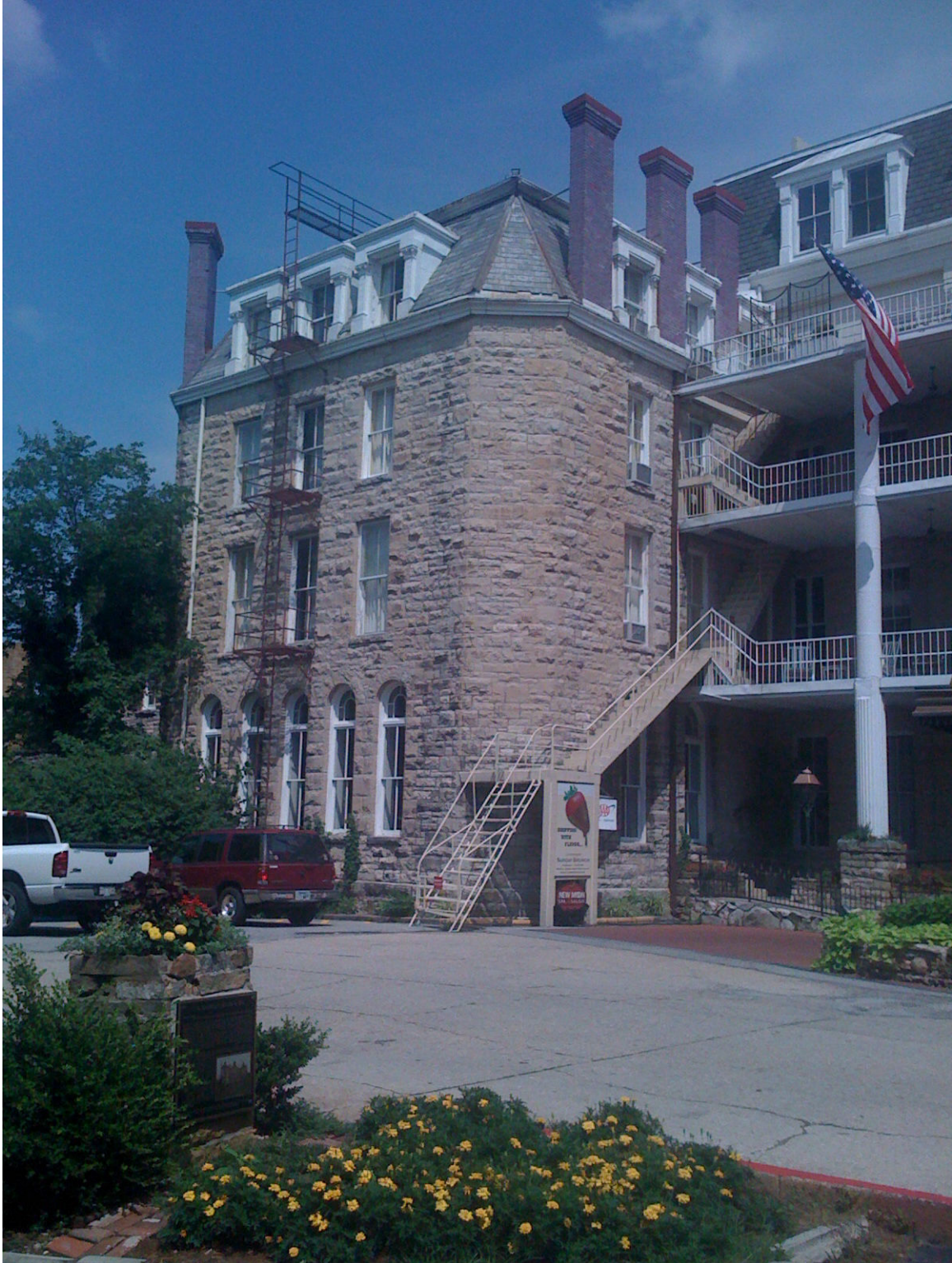
Part of the Crescent Hotel in Eureka
